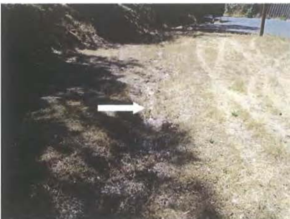
Photo 5. Rill erosion near Locust Avenue (arrow; 25 August 2009).
