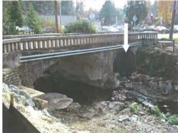
Photo 4. View looking at the west side of the Clay Street Bridge. Cedar Ravine joins Hangtown Creek via the culvert in the south abutment (arrow; 8 December 2008).
