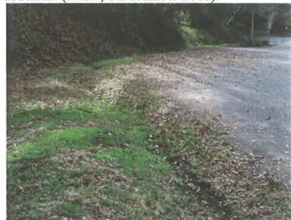
Photo 6. View of the roadside ditch along Locust Avenue (8 December 2008).
