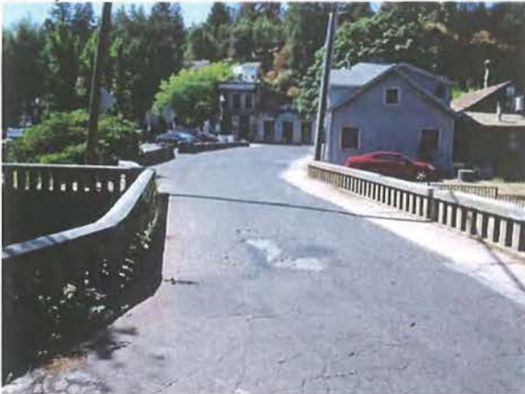
Photo 3. View looking south across the Clay Street Bridge over Hangtown Creek (25 August 2009).
